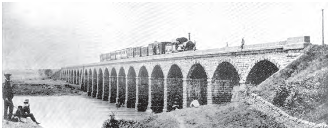
Fig. 1.4 First Railway Bridge linking Bombay with Thane, 1854
