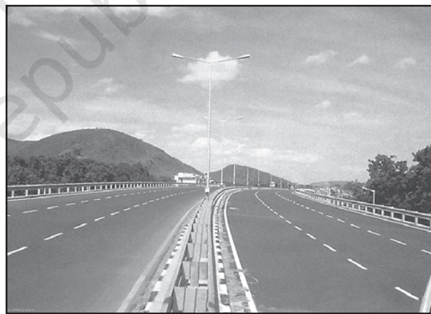
Fig. 7.3 : Dharmavaram Tuni National Highway, India
