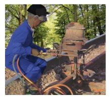
*Figure 3.11 Thermit process for joining railway tracks*  Can you identify the substances that are getting oxidised and reduced?
