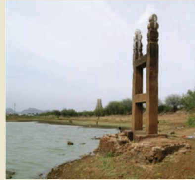
Sluice in Tank Srivilliputtur
